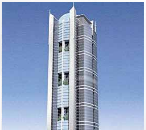
DUJA TOWER, DUBAI
