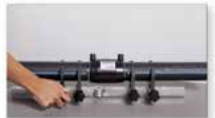
Clamps pipe and align it.
